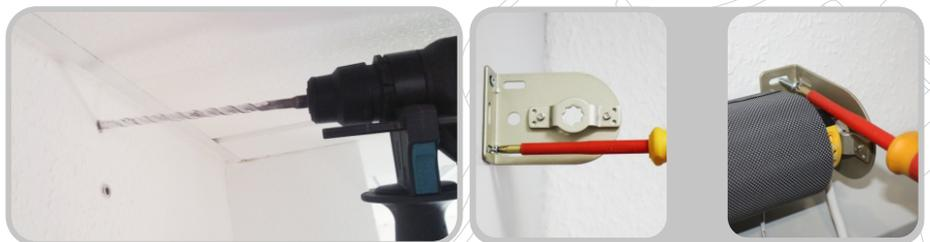
Measure the total width of the blind (including brackets), draw the height position of the brackets horizontally and mark the dowel holes. (or screw directly into wood for example)
